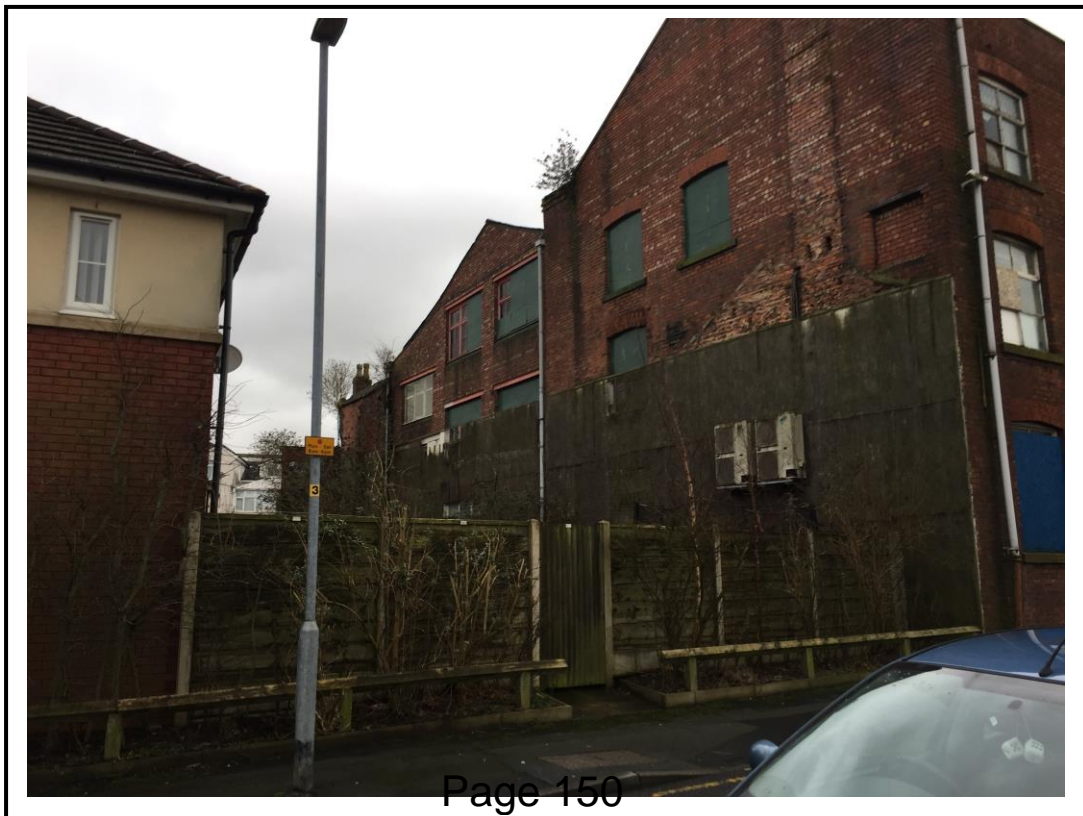
Photo 4 – view of buildings currently extending to the north eastern boundary of the site.
