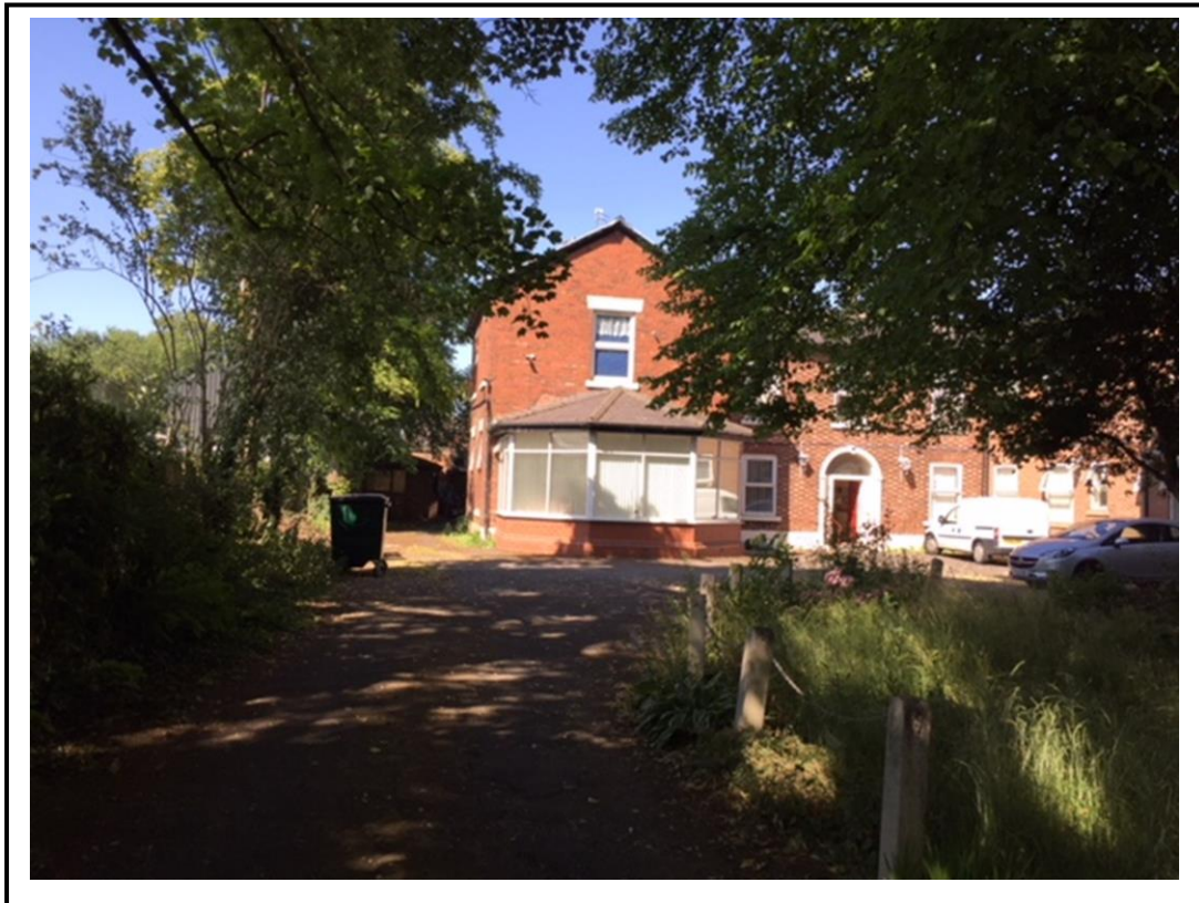
Photo 4 – view of existing building from entrance to the site
